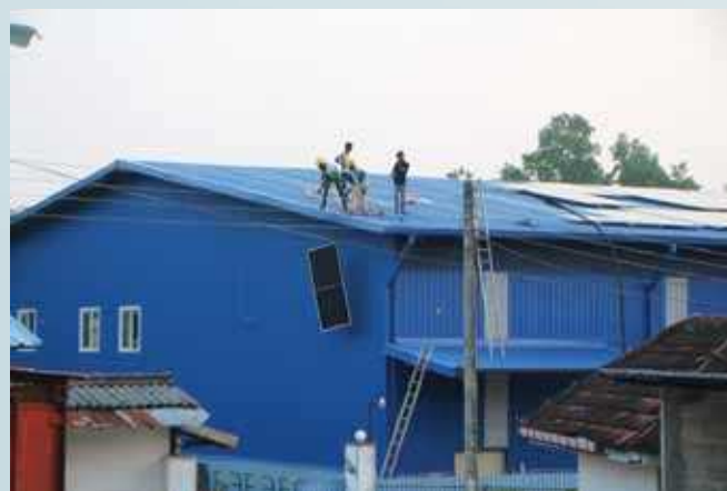
Installation of Solar panels
