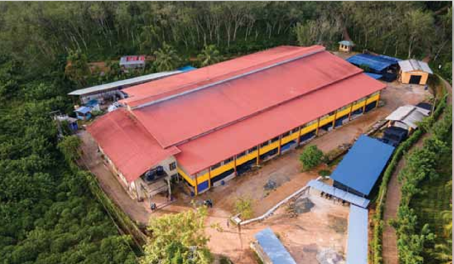
PVC Plant in Baddegama
